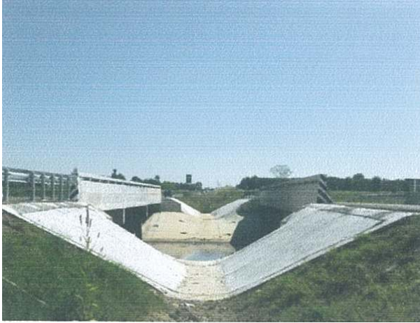
Concrete Slope Protection Km 13+123
